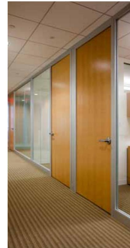
The offices of a large international foundation. The project features clear butt-glazed panels, 4" aluminum base trim and hinged full-height wood veneer doors. The door finish is quartered maple to match the furniture finish. The base trim and aluminum finish is "AC" Anodized Clear. Wide aluminum spacers are used at the end of GWB office dividing walls. The standard cylindrical locksets and the door hooks in satin chrome finish were chosen by the customer. Many hardware options are available.
